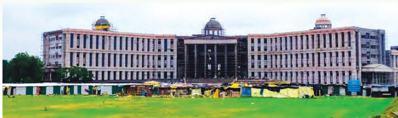
Academic Block under construction
