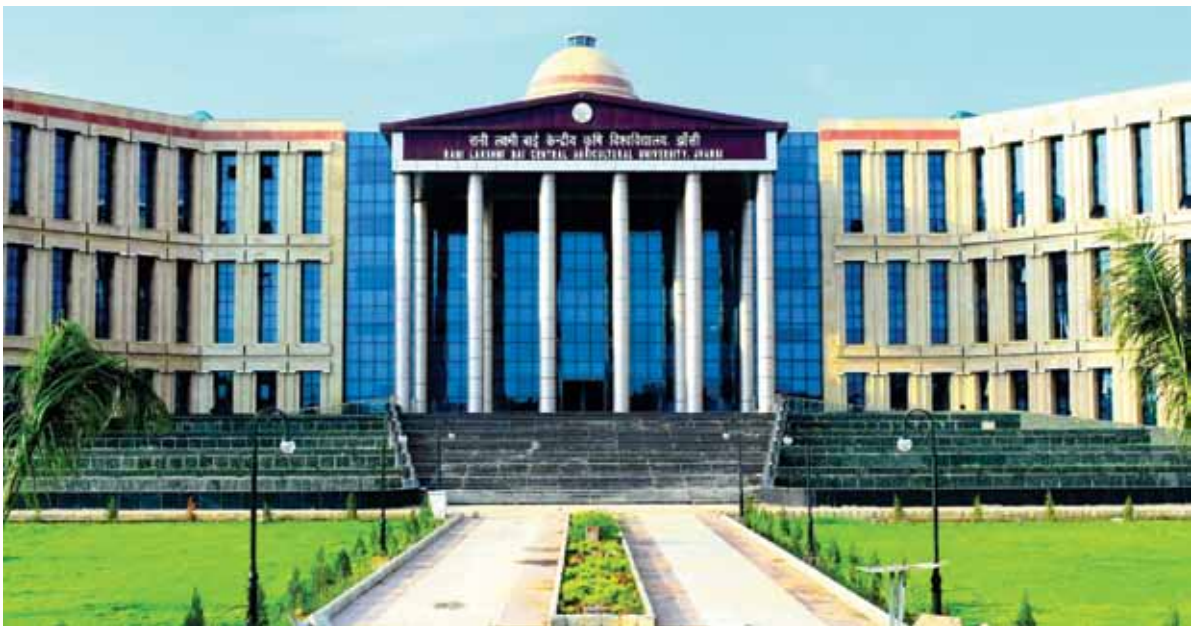
A glimpse of newly constructed Academic Building
