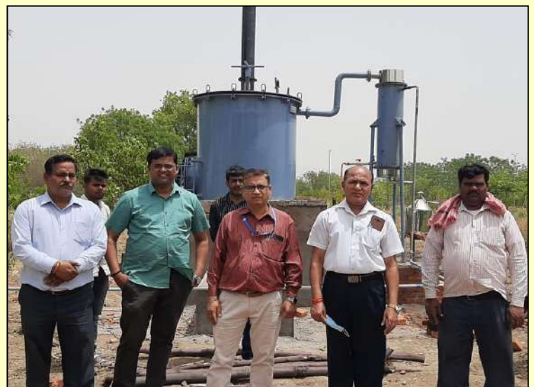
Fig. 1: Fig: Installation of Grass Oil Distillation Unit
