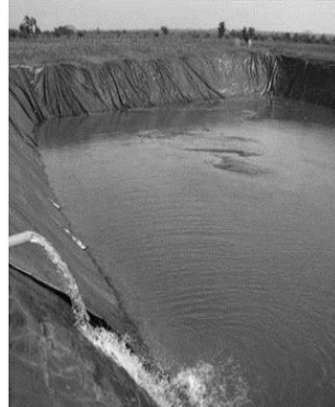
Construction of pond for irrigation
